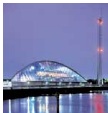
Glasgow Science Centre from the Clyde (David Barbour / Building Design Partnership)
